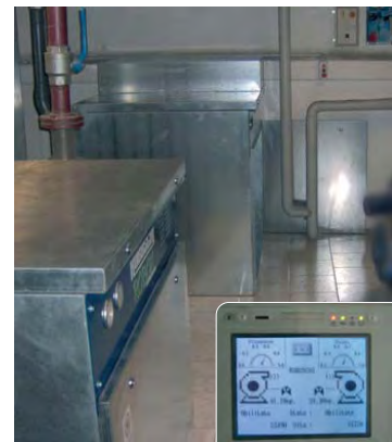
• Paper industry: Centralised vacuum systems ROBOX evolution pressurised blower unit in pressure (P) / air injection vacuum (DV)
