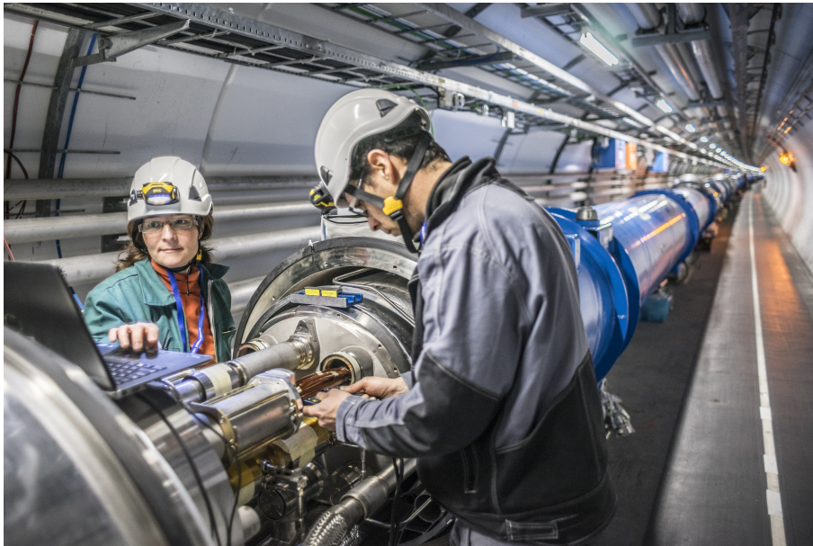
Figure 1.1.1: Workers at the tunnel during long shutdown [2]
