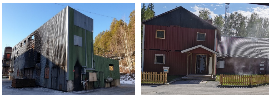
Figure 3. A building (left) used for LS, representing, e.g., a four-story apartment building, a mechanical workshop or a cruise ship, depending on the selected scenario. A family house with an attached garage (right), where the fire in the garage can only be represented by generated cold smoke, thus not behaving as a corresponding real fire.
