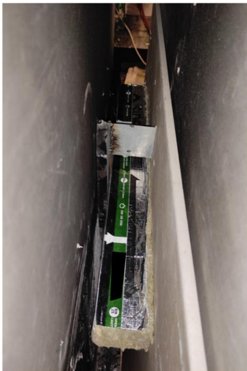
Figure 29 – The cavity barrier installed with an L steel angle in front.
