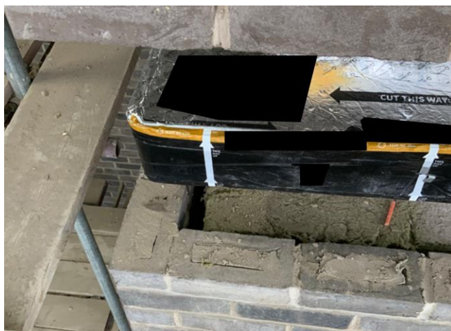
Figure 87 - Deviation from the installation guidelines noticed for the corners
