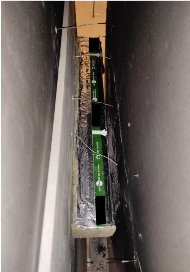
Figure 35 –The cavity barrier blocks installed for the scenario 6.
