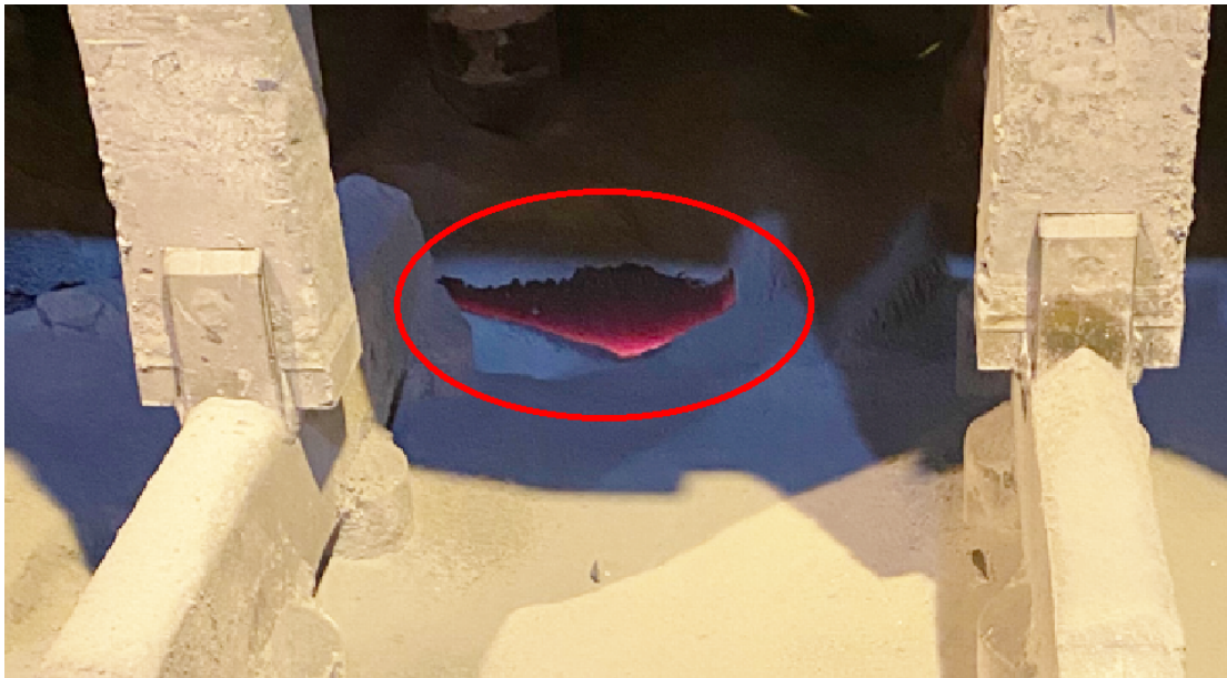
Figure 1.2.1: Inside an electrolysis cell: a hot spot on an anode.
