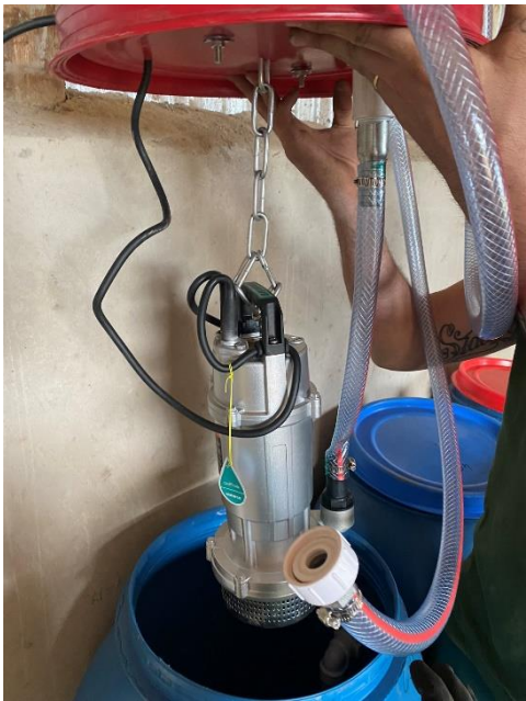
Picture 20 - Water Pump in T4 Plastic Sieve in T1 (Langseth, 2023)
