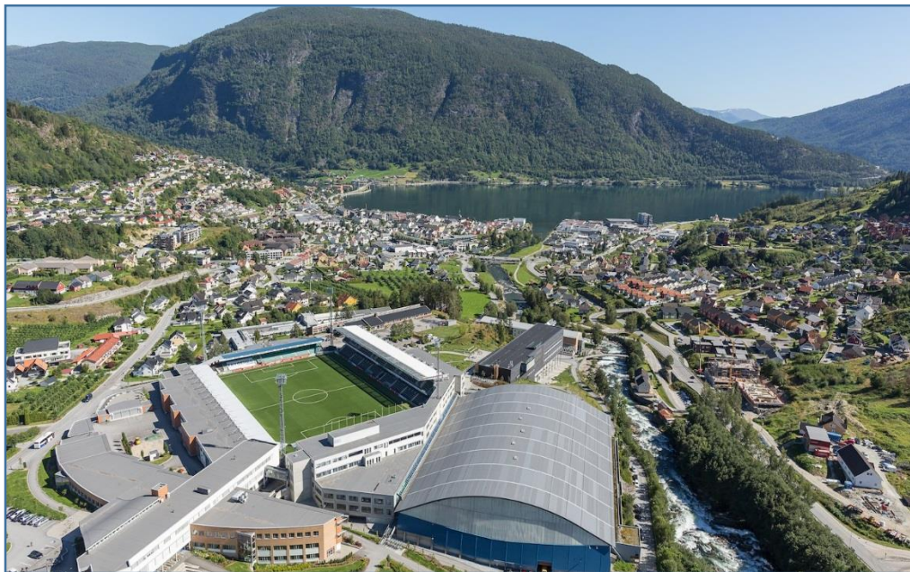
Fig 3: Aerial view of pitch of Fosshaugane Campus Stadium ( Fosshaugane Campus, 2016 )
