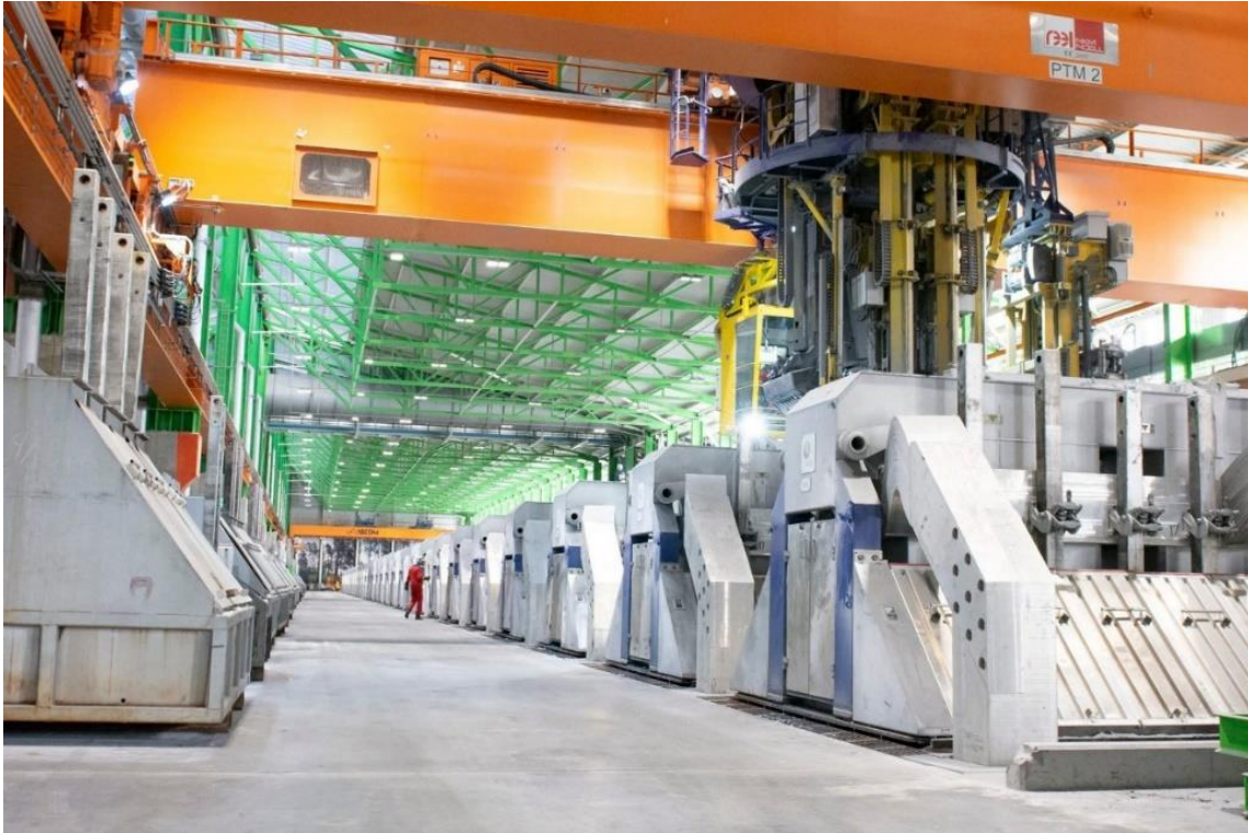
Figure 11 - Karmøy Technology pilot. (Hydro, 2020).
