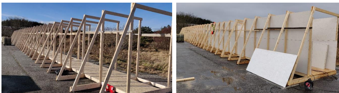
Figure 16: Construction of the corridor in ResQ safety centre
