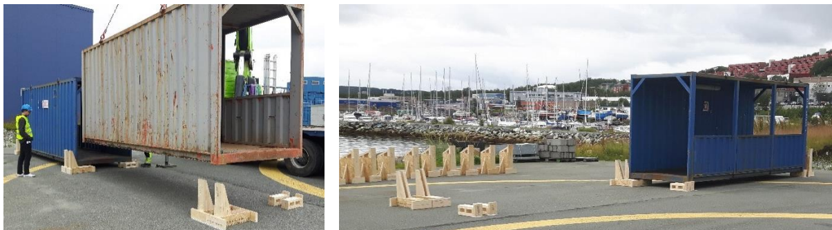
Figure 13: Rigging the container corridor on 0° legs at Arcos safety centre
