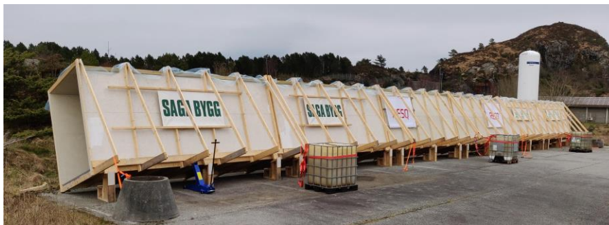
S3: The Haugesund test facility heeled at 20°
