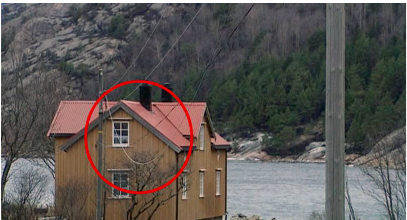
Fig. A3. The fire was caused by sparks from an aluminium power line, with a detached upper cable striking the lower cables in strong wind. The sparks ignited cured grass. (Photo: NRK, reproduced with permission.).
