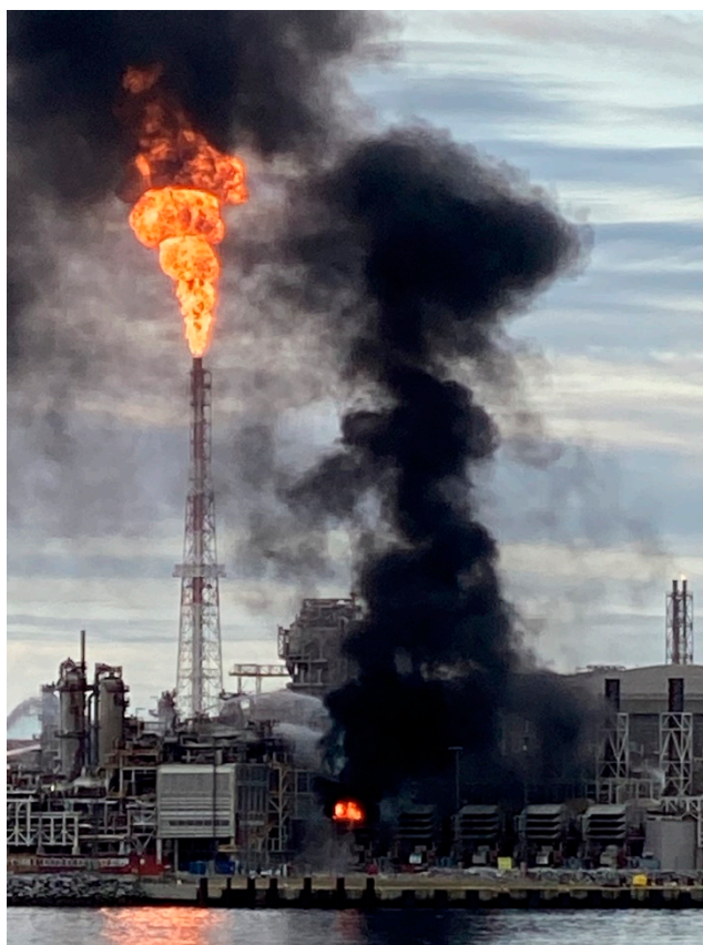
Figure 17. Photo of the GTG 4 air intake fire with the process depressurization flare in the background. Photo by Stein Lyder taken from Sørøysundekspresen. (Reproduced with permission.).
