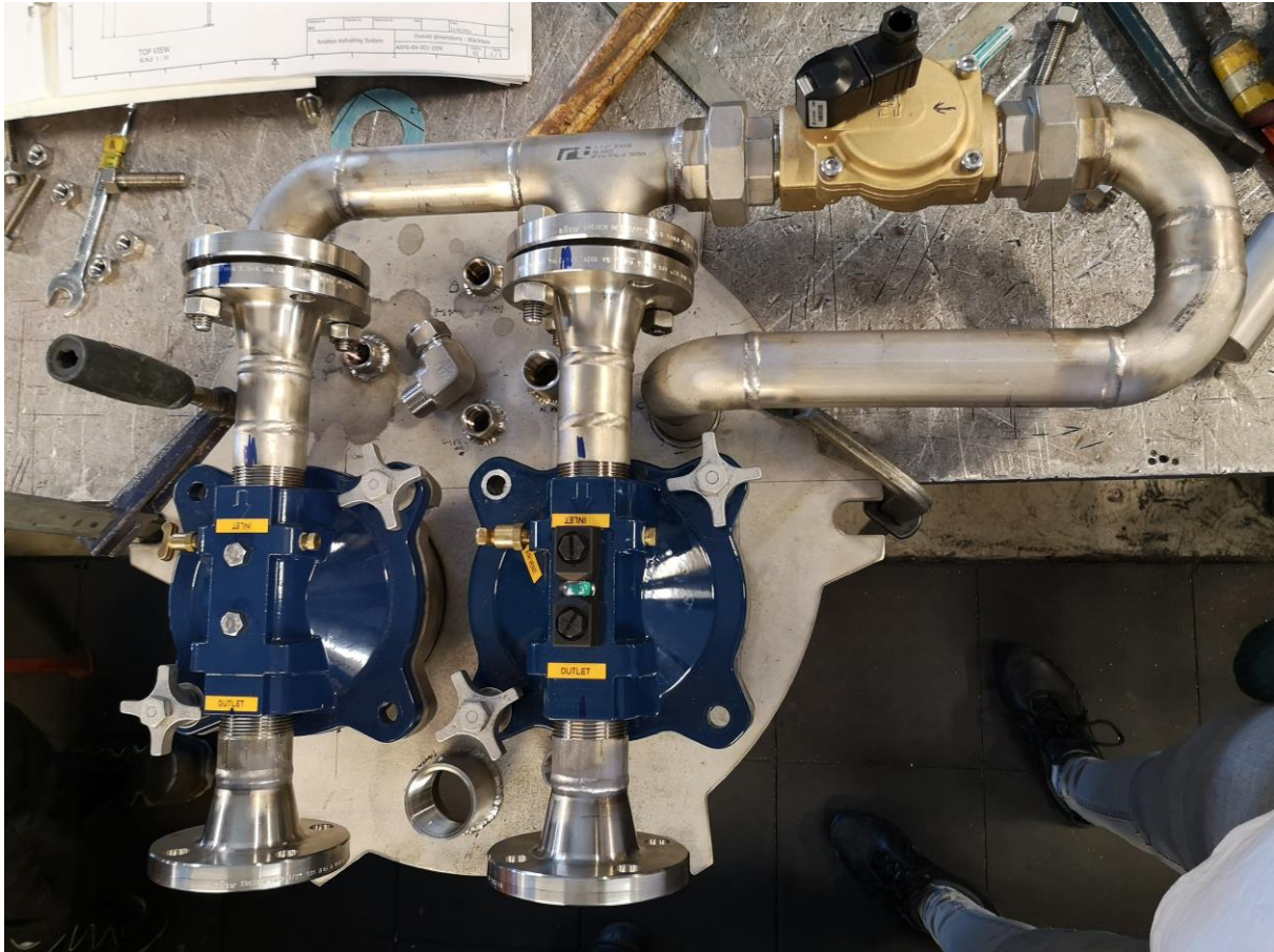
Figure 3.14 – Tank lid with filters in building process
