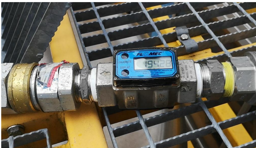
Figure 4.14 – Master flow meter during testing
