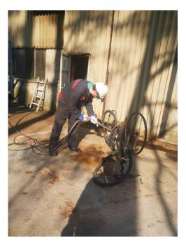
Figure 36 - Using Oxyacetylene torch
