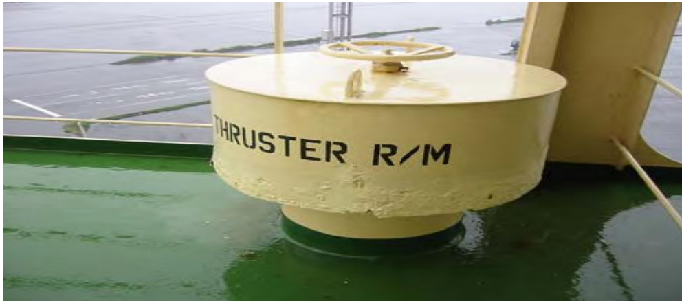
Figure 2.6: Wastage of the casing of ventilator
