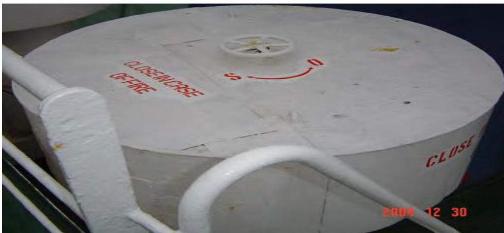
Figure 2.7: Temporary repair by tape
