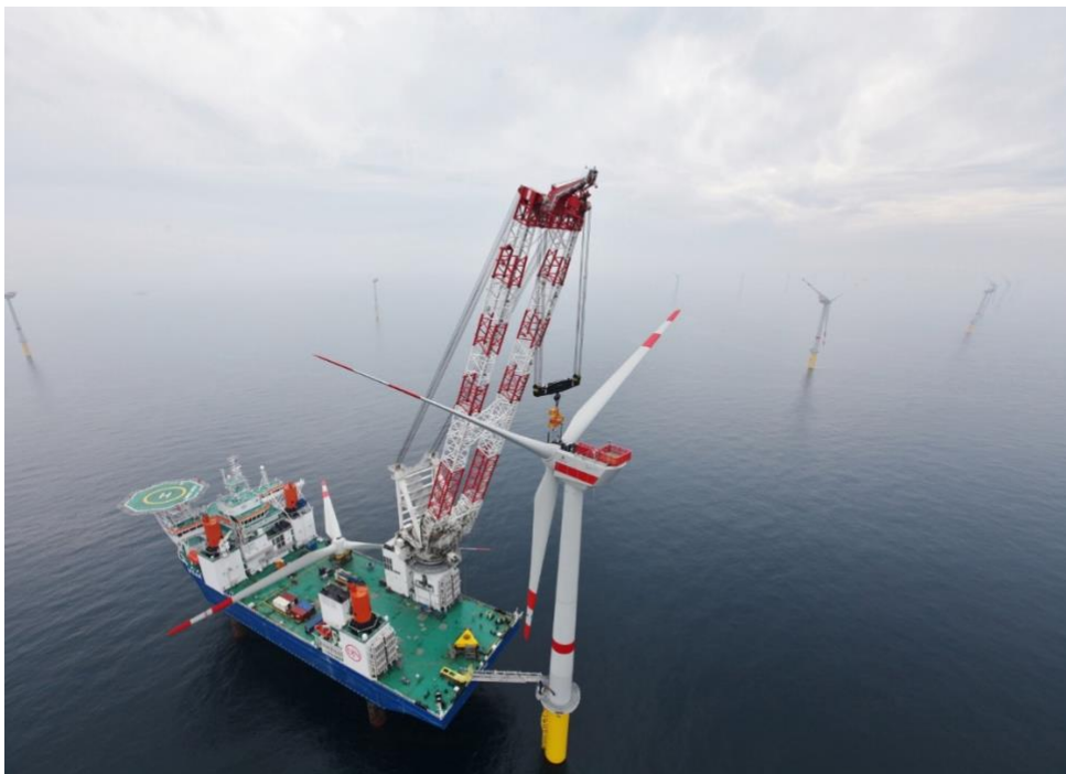
Fig. 22 offshore jack-up crane vessel Vidar installation of an OWT, from [56]
