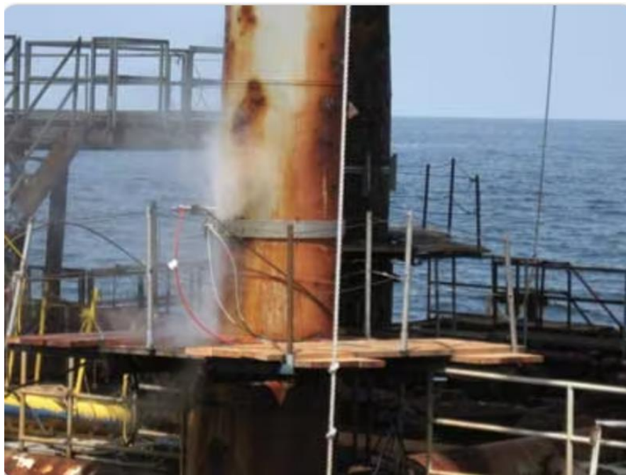
Fig. 32 Top side application of AWJ, from [67]
