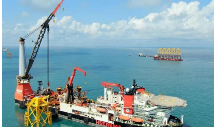
Fig. 25 HLV Aegir installing a jacket foundation, from [56]
