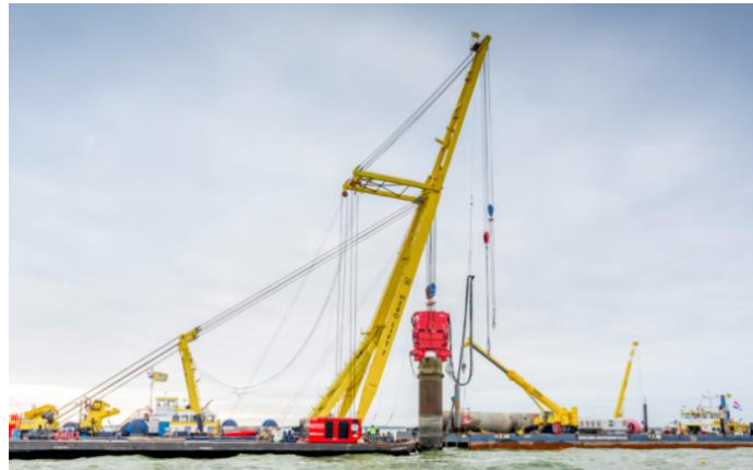
Fig. 17 Decommissioning of Lely offshore wind farm foundations, from [44]
