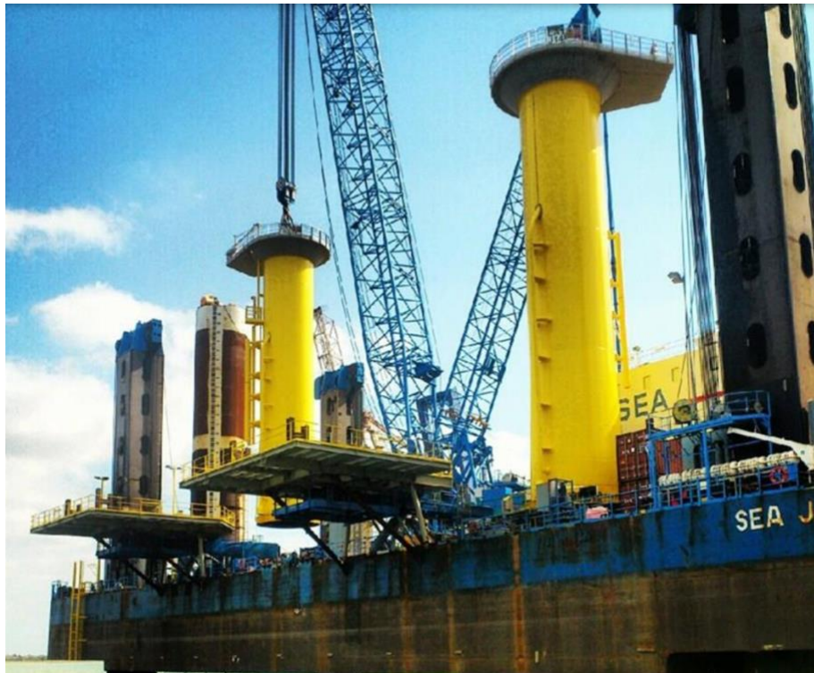
Fig. 27 Sea Jack lifting and transporting OWT foundations, from [62]
