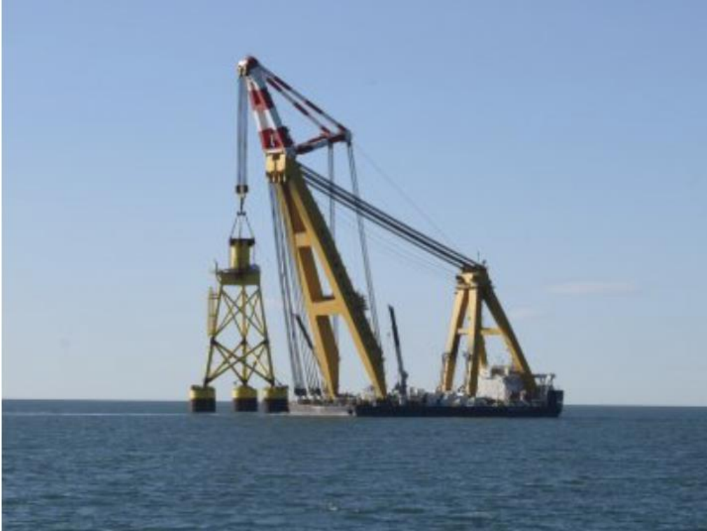
Fig. 4 Installation of jacket foundation for Aberdeen Offshore wind farm, from [23]
