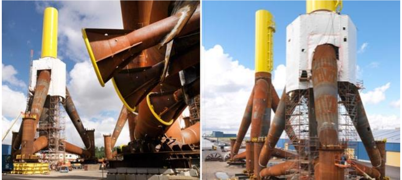
Fig. 3 Tripod foundations for Global Tech I., North Sea, Germany, from [21]
