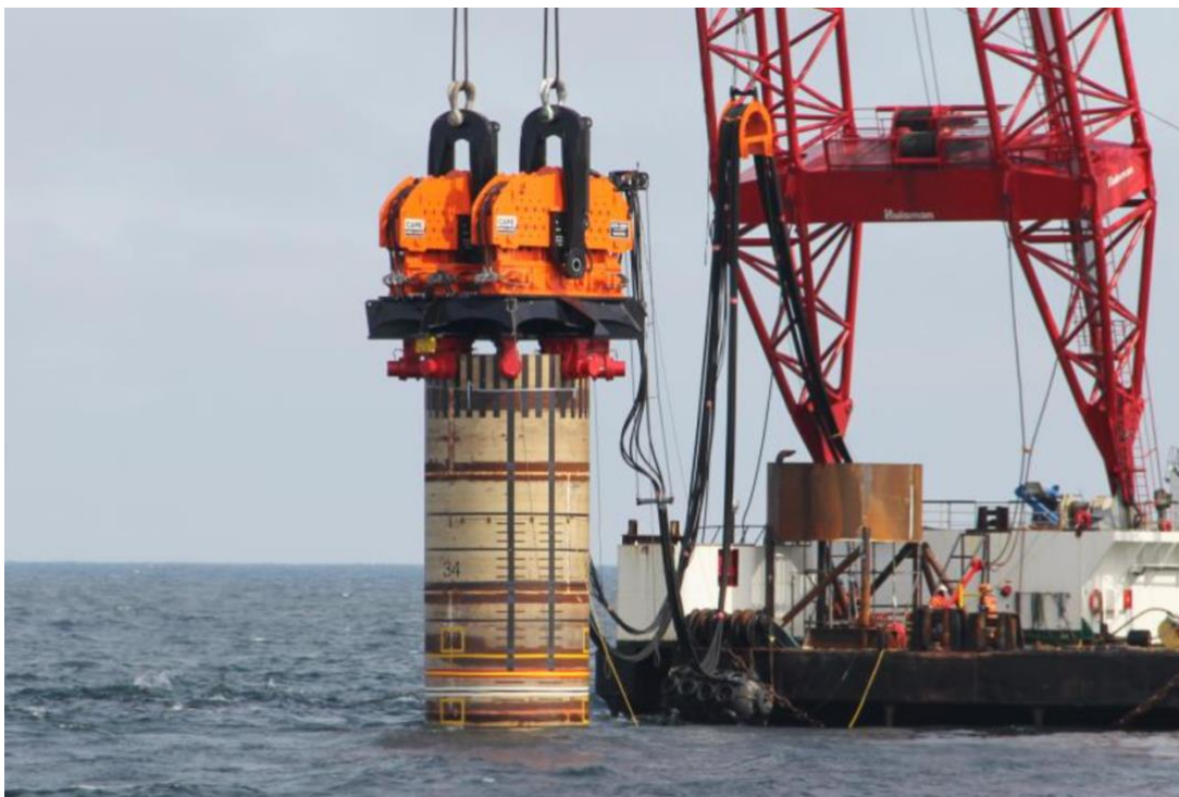
Fig. 40 Vibrator on an offshore monopile, from (Wassink, 2018)
