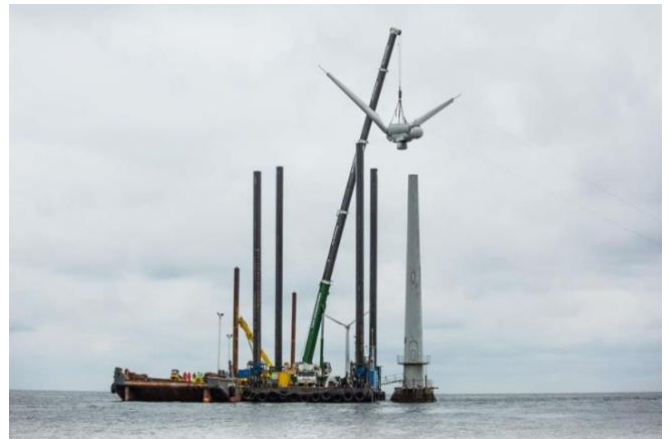
Fig. 18 Decommissioning of Vindeby wind turbine, from (Weston, n.d.)
