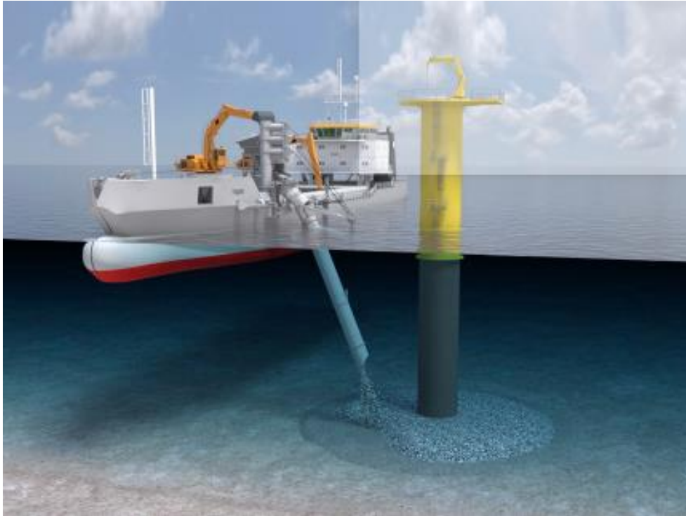
Fig. 15 Scour protection after the monopile (seen in gray) and transition piece are installed, from [43]
