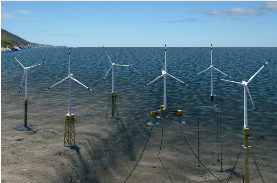
Figure 2 - Offshore wind substructures
