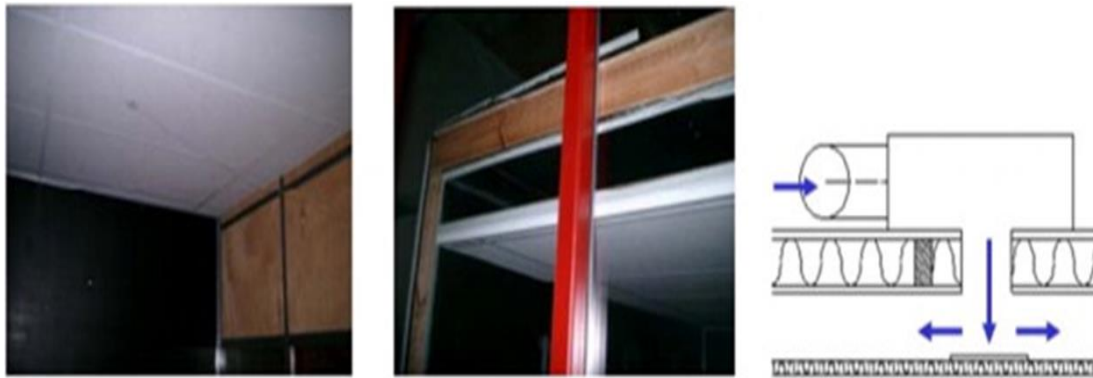
(a) Room with diffuse ceiling inlet (b) Location of ceiling panel (c) Supply opening to the plenum
