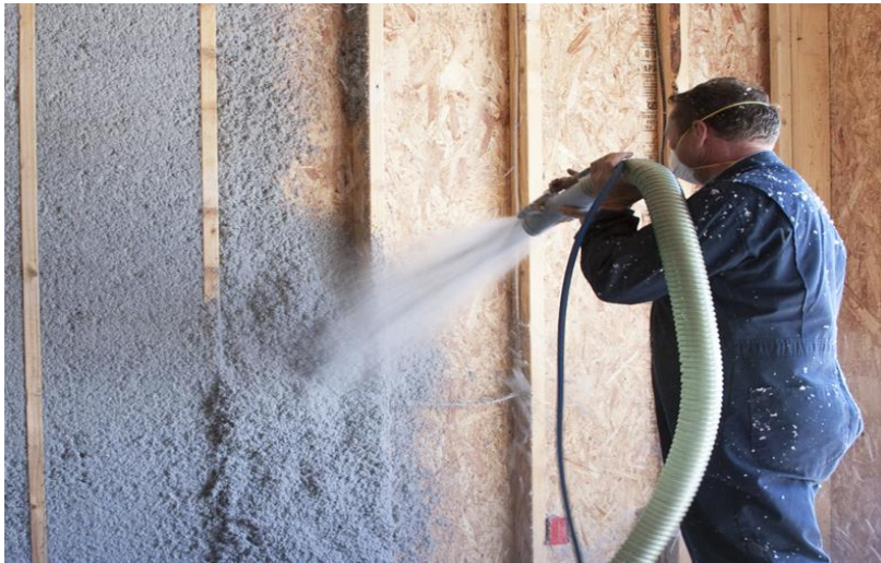
Figur 25 Cellulose sprayes mot en vegg (Mlive Media Group (2011).
