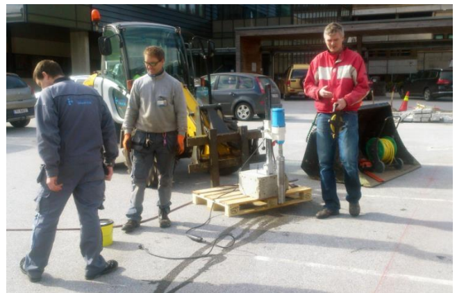
Figure 10: Installation in progress
