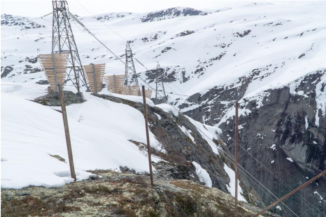
Figure 3-12: The snow cover had been notably reduced by 05.05.20. Note the bare ground around the closest baffle.
