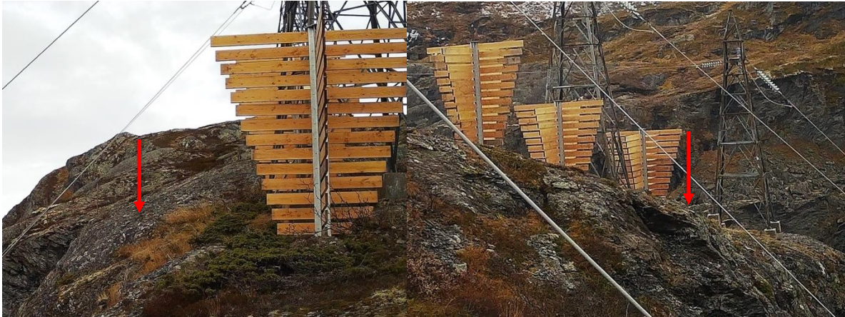
Figure 4-3: Images from Cam 1 and Cam 3 showing the position of the rocky outcrop (red arrow) ridge ward of baffle 3 and 4. A small cornice developed at this location during the monitoring period.
