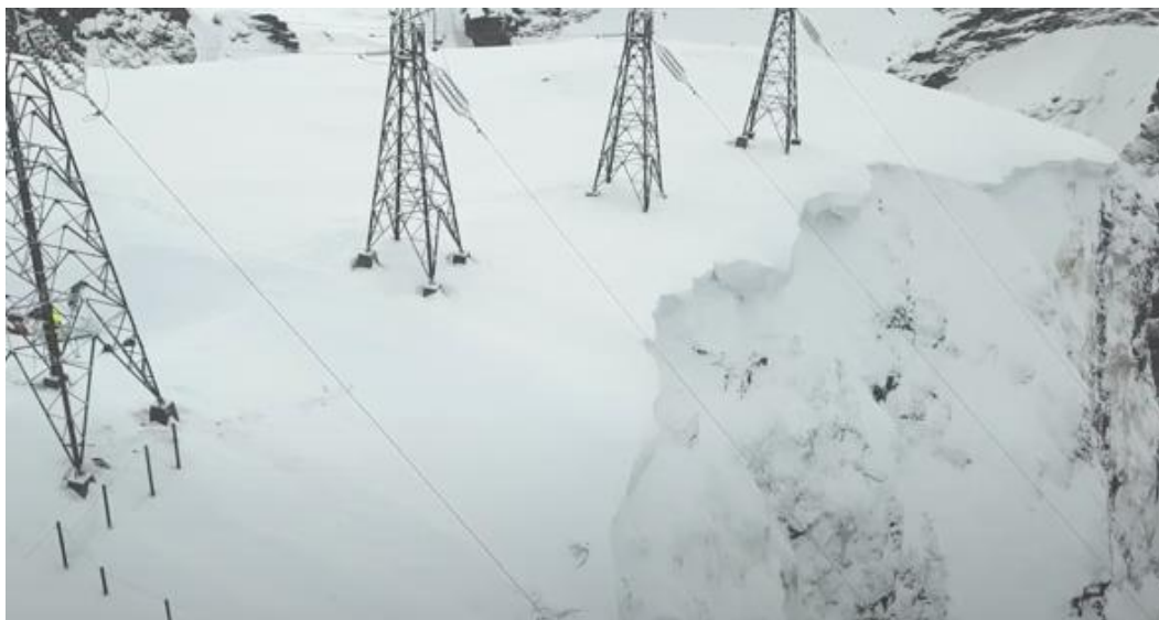
Figure 3-20: Aerial image before explosive work was conducted 21.02.2018. A long continuous cornice had developed along the ridge and the powerline on mast 2 had come in contact with the snow.
