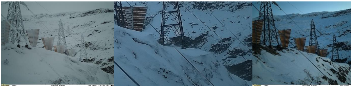
Figure 3-5: The first accretion event could be seen 14.12.19 (pictured in the middle). A cornice developed in the reference area as well as on the outcrop between baffle 3 and 4. Images from Cam 2. From the left: 10.12.2019, 14.12.2019, 22.12.2019
