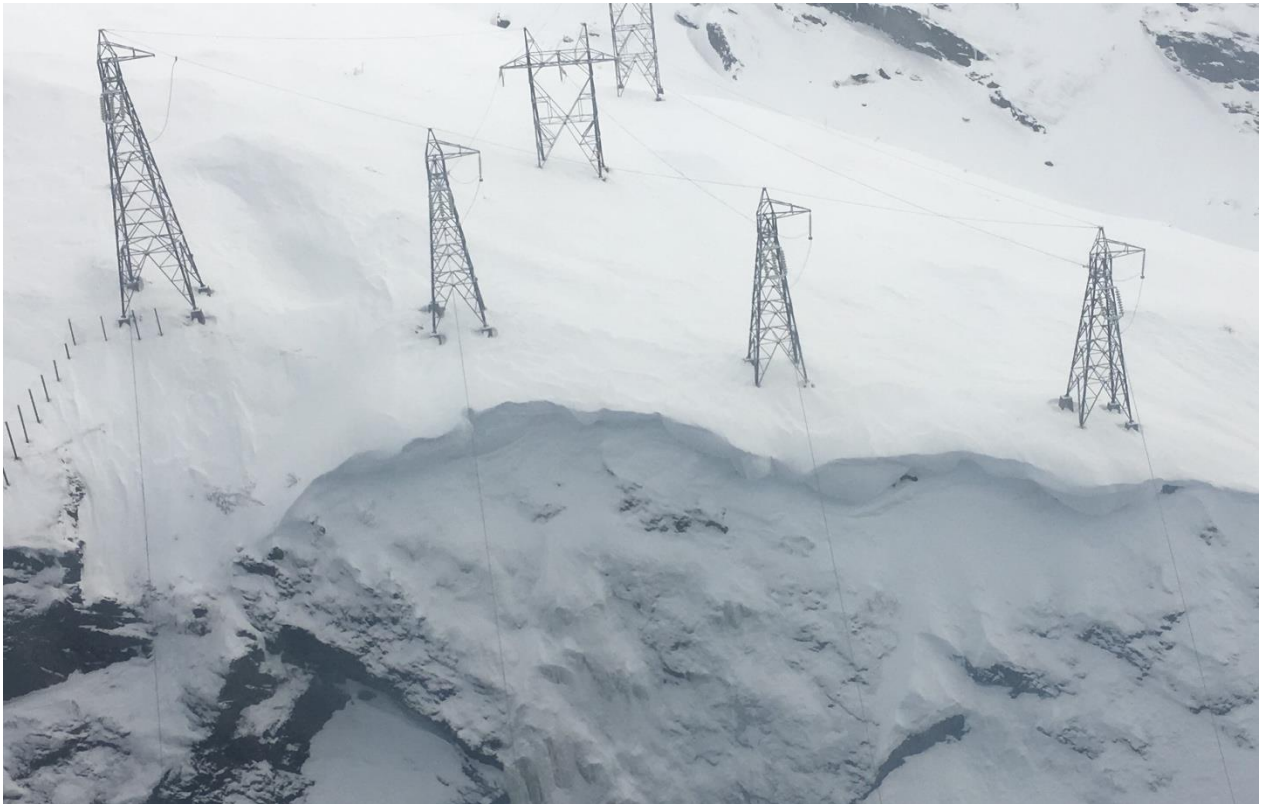
Figure 1-1: The horizontal extent of the cornice structure at Kvannberget has previously interfered with the power lines. Note the small depression at the lip of the cornice where the powerline from the second mast from the left was in contact with the snow. The image is from 2018.
