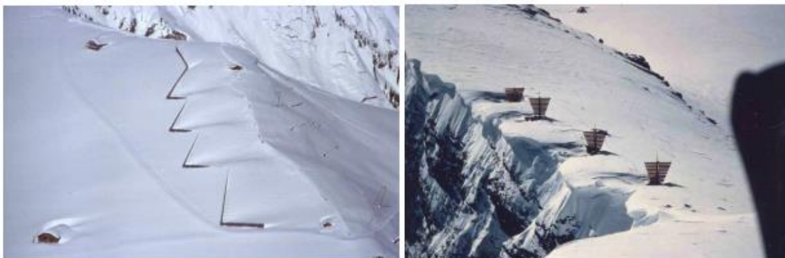
Figure 1-3: Snow fences to the left and wind baffles to the right (Hákonardóttir et al., 2008). Note the increased deposition around the snow fences and the increased erosion around the wind baffles.
