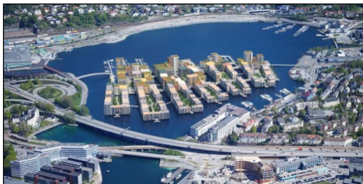
Figur 1 Trenezia (Waugh Thilstleton Architects)
