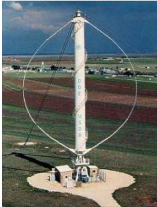
Figure 2-2. Experimental Department of energy (DOE) and US Department of Agriculture (USDA) 34-meter diameter Darrieus Wind turbine [7]
