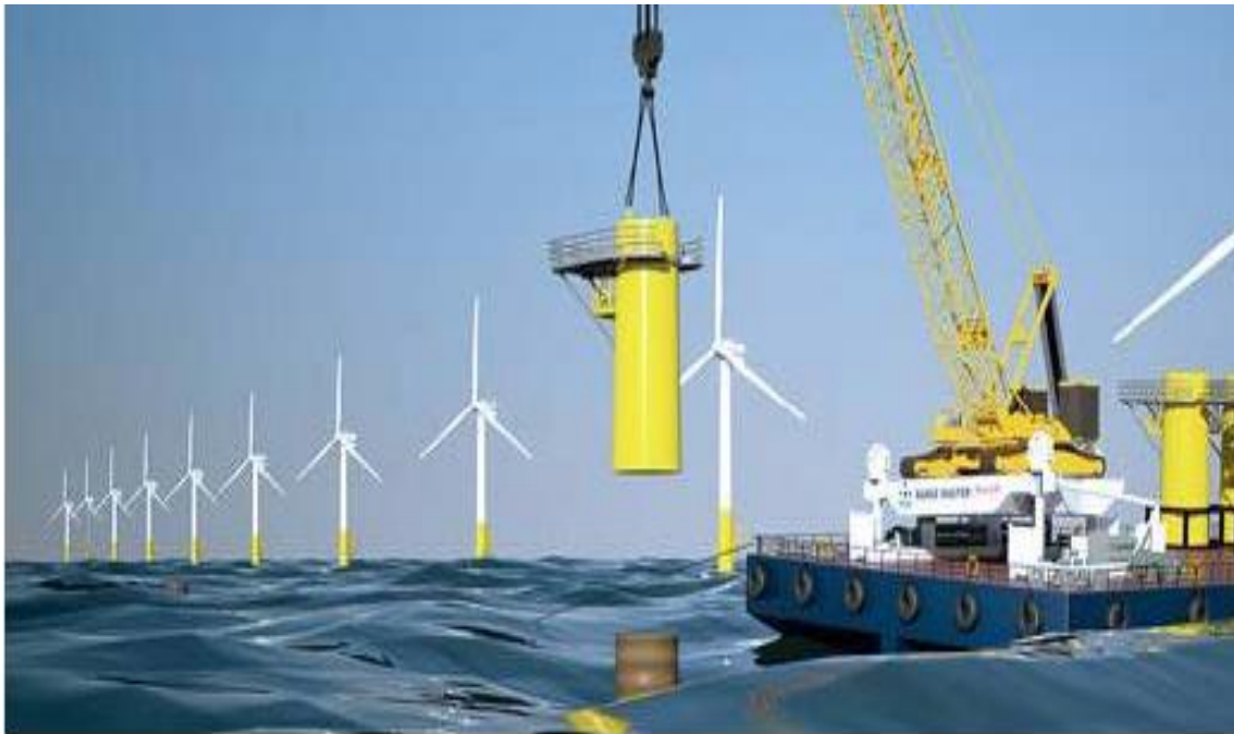
Figure 34 Heave Compensated Barge Installing a Transition Piece (Kopits and Losz, 2013).
