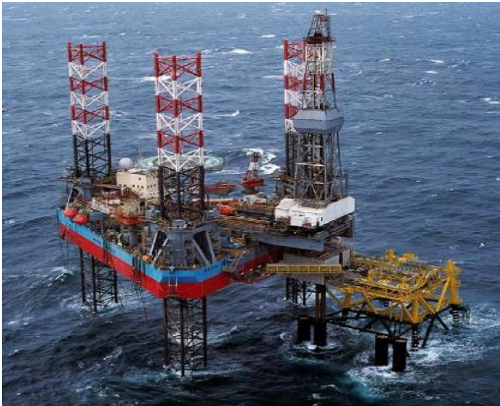
Figure 10 Jack-Up Rig (Energy Endeavour, 2008 as cited in Bay & Bai, 2012)
