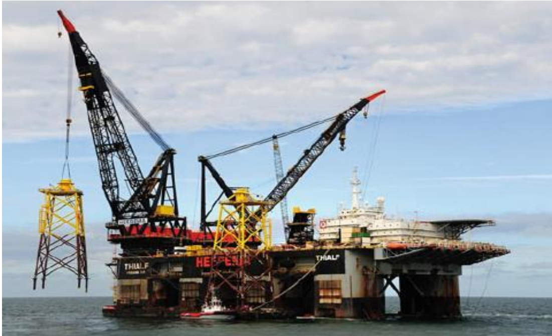
Figure 22 Alpha Ventus foundation installation (Alpha Ventus,2010 as cited in Kaiser & Snyder, 2012)
