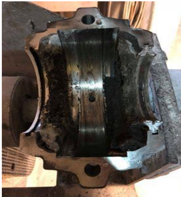
Figure 5. 10: Bearing house full of contaminated grease
