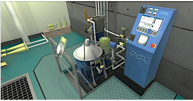
Figure 5: The fuel oil separator system of the immersive VR simulator
