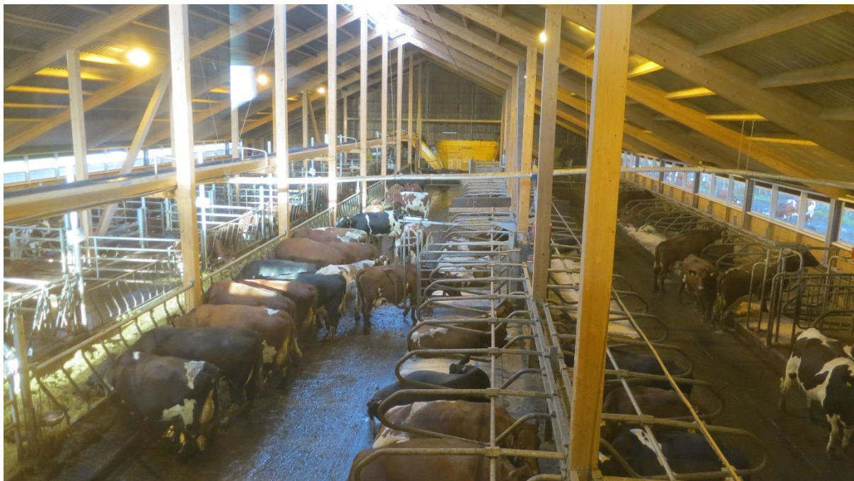
Figure 7: Ceiling panels on barn roof.
