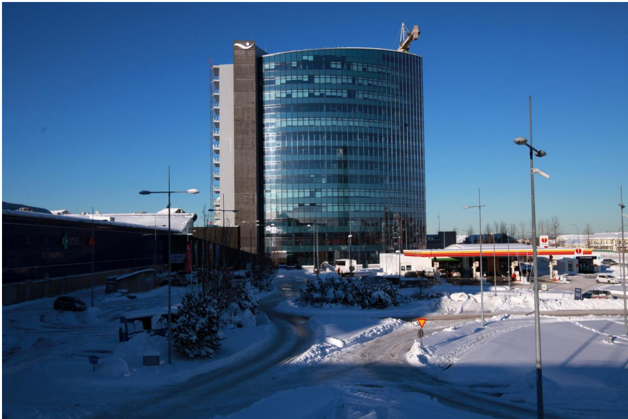
Figure 15: Picture of Norðurturn 3
