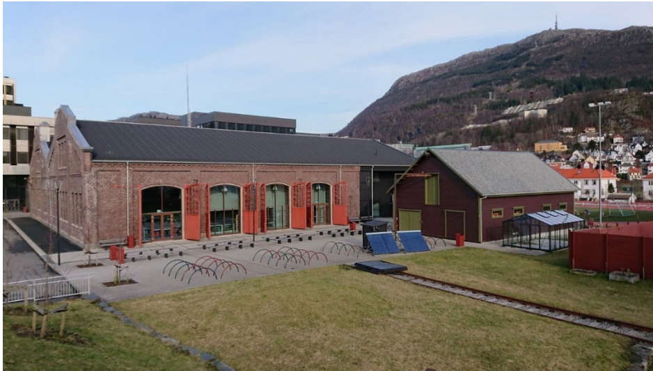
Figure 1 Solar laboratory site, January 2019
