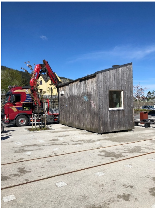
Figure 21 The passive house in its final position
