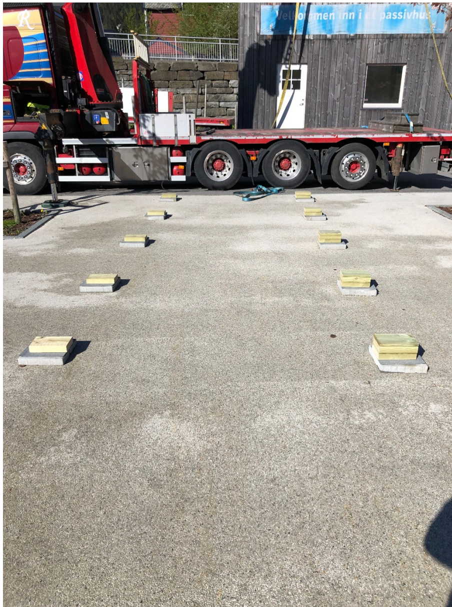
Figure 16 Foundation blocks laid out before the house were placed onto them
