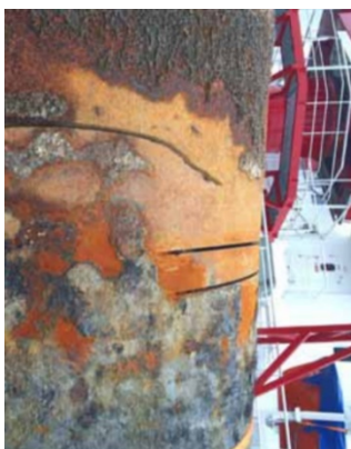
Figure 32 - Diamond Wire Cutting attempt not Successful on Vertical Pile [61]
