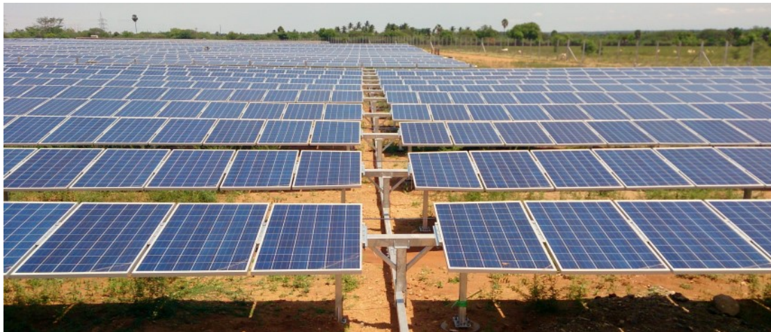
Figur 5 Horizontal single axis trackers i Vellakoil, India (Wikipedia, 2014)
