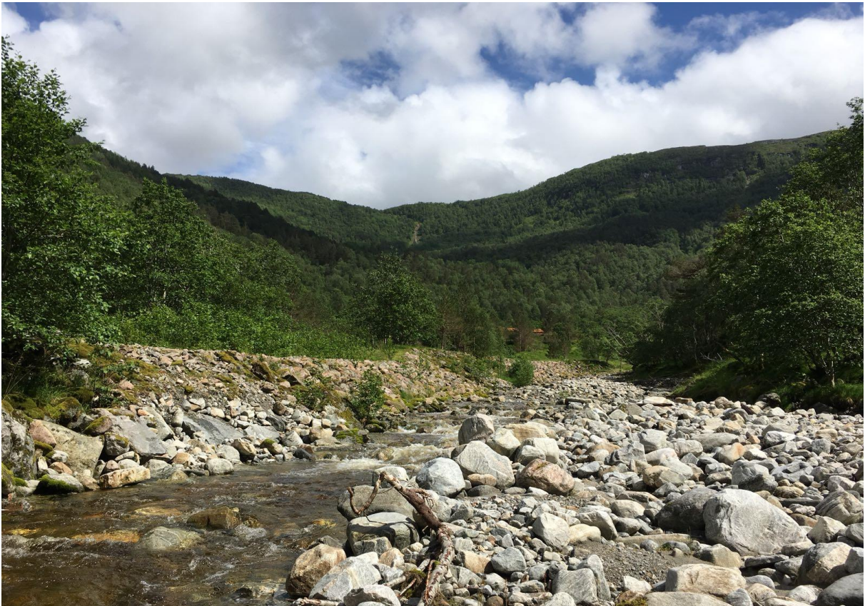
Figure 3.8: Flood protection Øystrebølva, showing the elevated riverbank on the left (Paetzel, 2017b).
