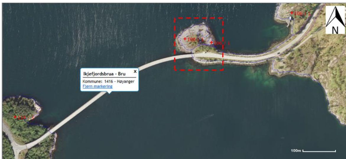
Figure 3.9: The Ikjefjordsbrua. former island Storeholmen is indicated in a red striped square (kartverket, 2018).
