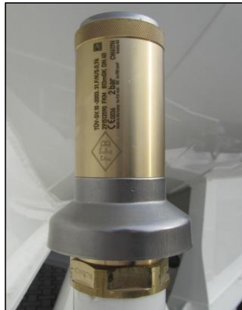
Picture 6: Safety valve
