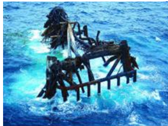
Bilde 3 Mumbai High North etter kollisjonen med Samundra Suraksha. Hentet 01.05.16 fra: http://www.mace.manchester.ac.uk/project/research/structures/strucfire/images_export/CaseStudy/HistoricFires/Other/platformDestroyed.gif
