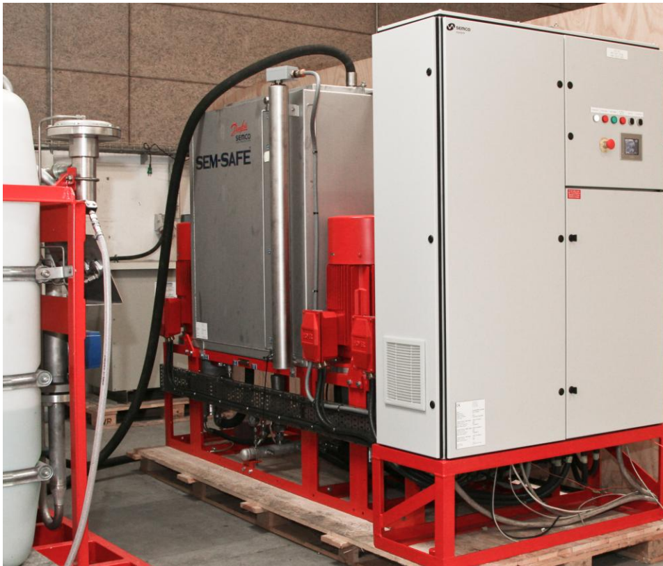
Figur 7 Sem-Safe Water Mist pumpeenhet
