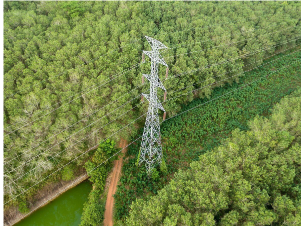
Fig. 1.1: Transmission tower and relative power line corridor in a forested area. Image from [179].
