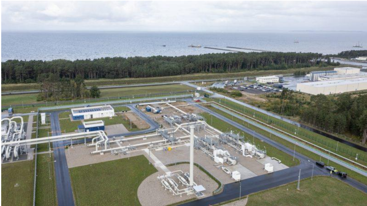
Figure 3: Gas receiving terminal [2]
