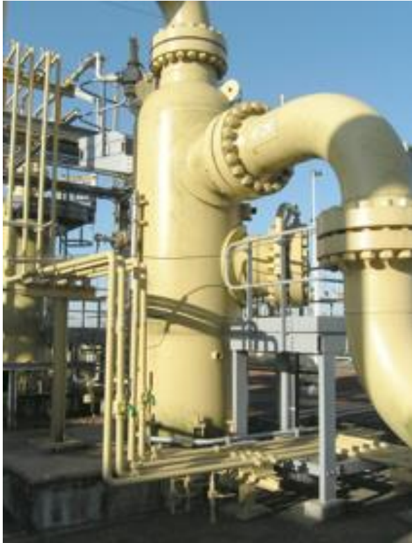
Figure 5: Existing cyclone separator [2]
