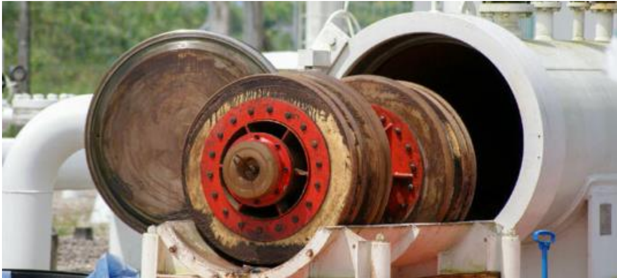
Figure 9:Pig entering pipeline [17]
