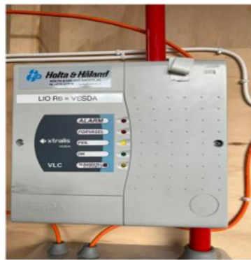
Figure 9: Components of the fire alarm and detection system
