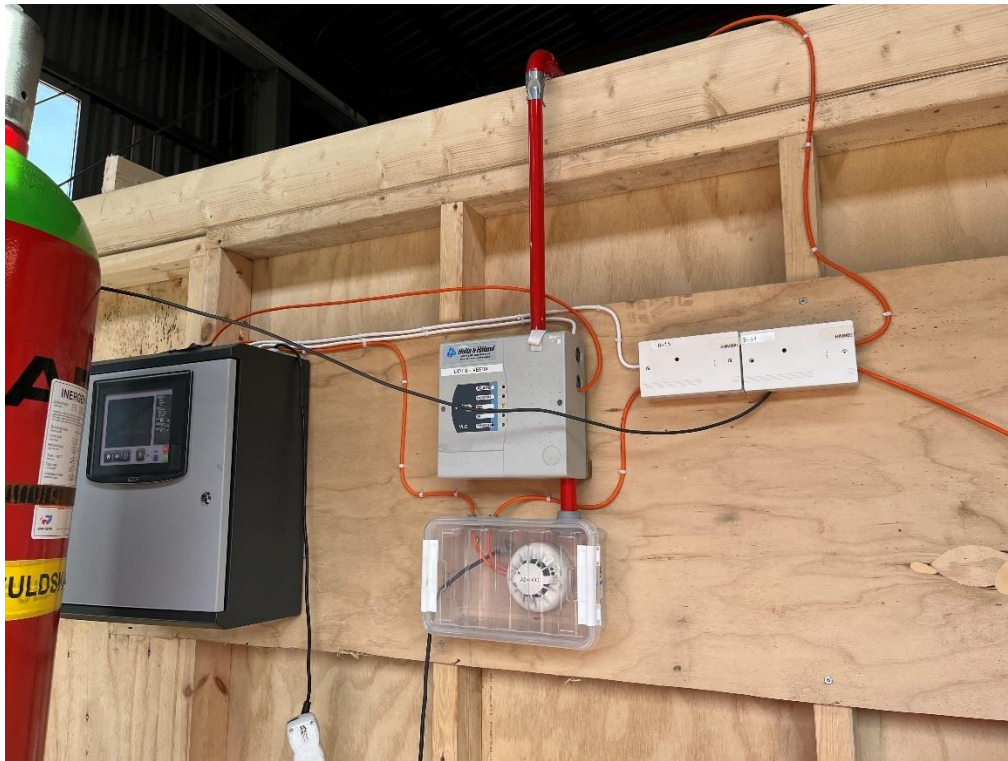
Figure A3: Boxed chamber of multi-sensor detector at the exhaust of aspiration detection Unit
