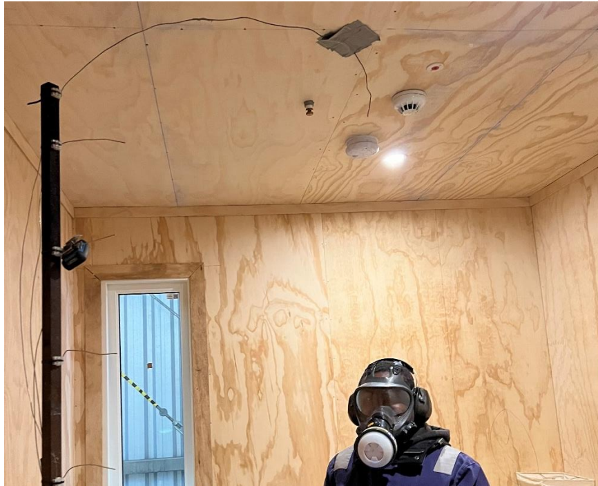
Figure A5: Bedroom of apartment showing thermocouple stack-3, smoke detectors and volunteer participant during test with activation of inergen gas extinguishing system
