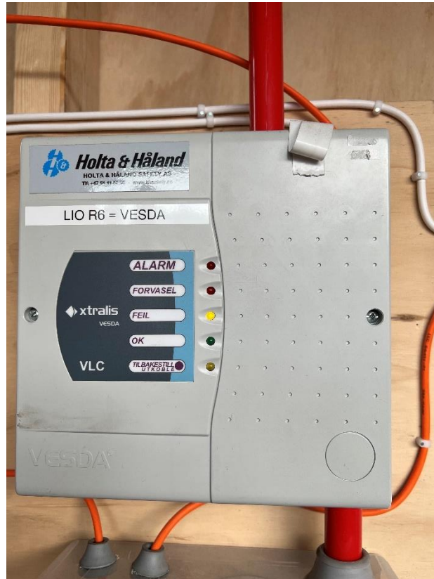
Figure A9: Aspiration Detection Unit and control panel
