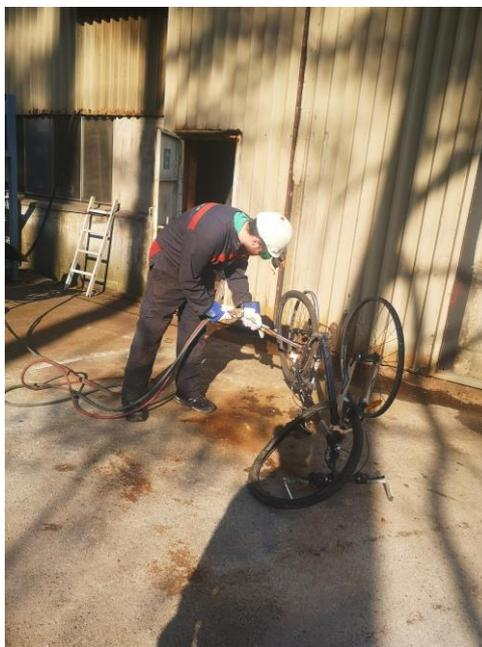
Figure 36 - Using Oxyacetylene torch
