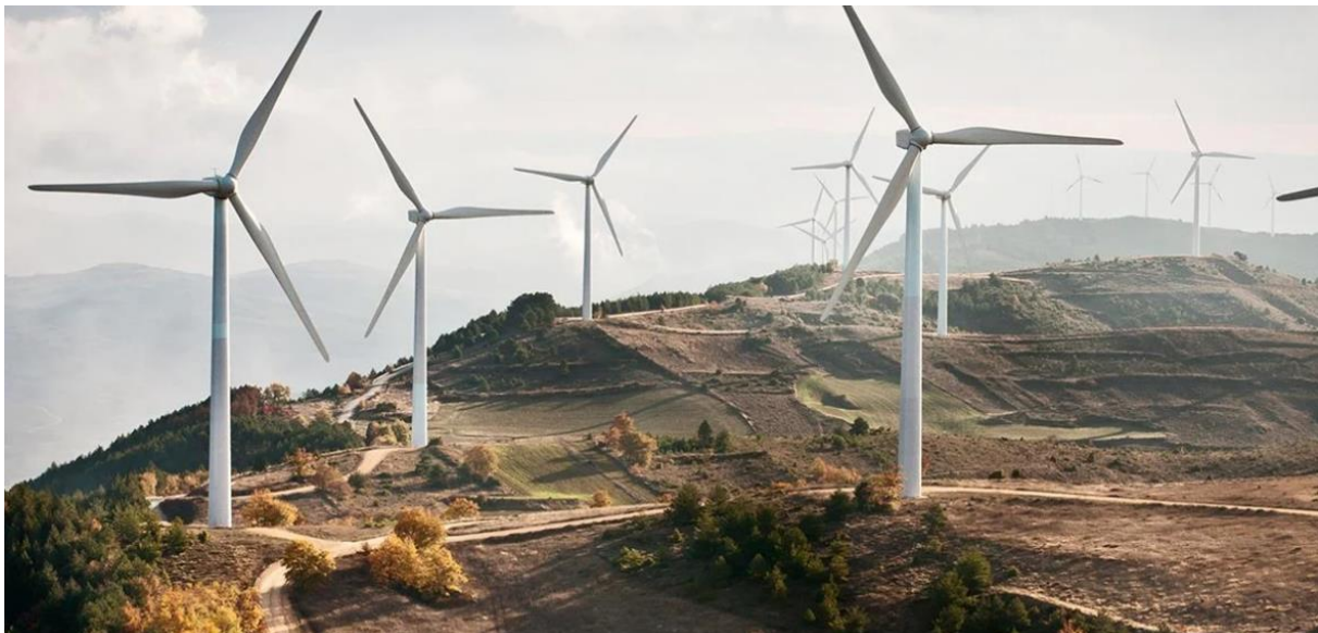
Figure 2-6. Onshore wind farm example, source [Roxtec Global, 2013]
