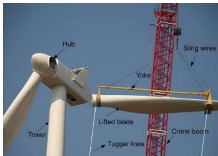
Figure 3-3. Blade assembly, source [Power Technology, Lake winds energy parks, Mason County, Michigan, 2017]
