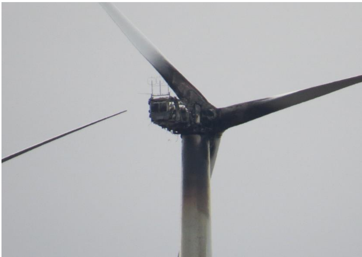
Figure 4-3. Norway Fitjar Midtfjellet Vindkraft turbine fire, source [Haugesund Avis, 2015]
