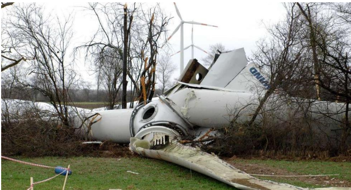
Figure 2-19. An example structural failure of onshore wind turbines, source [Tallbloke's Talkshop, 2014]
