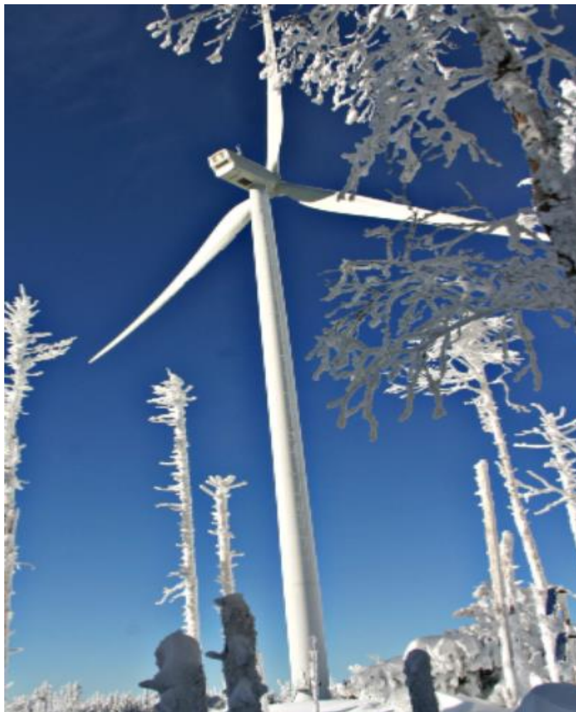
Figure 4-4. The wind turbines above the Balsams, source [IndepthNH, 2016]
