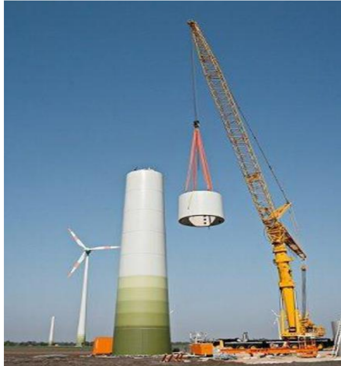
Figure 3-2. Tower assembly, source [Betontec, Clean Energy Structures, 2019]
