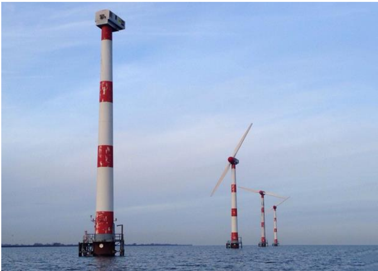
Figure 4-2. Wind turbine blades fell in Netherlands, Lely Wind Farm, source [National Wind Watch, 2014]
