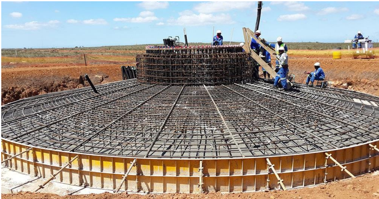
Figure 3-1. Wind turbine foundation work, source [Creamer Media's Engineering News, 2014]
