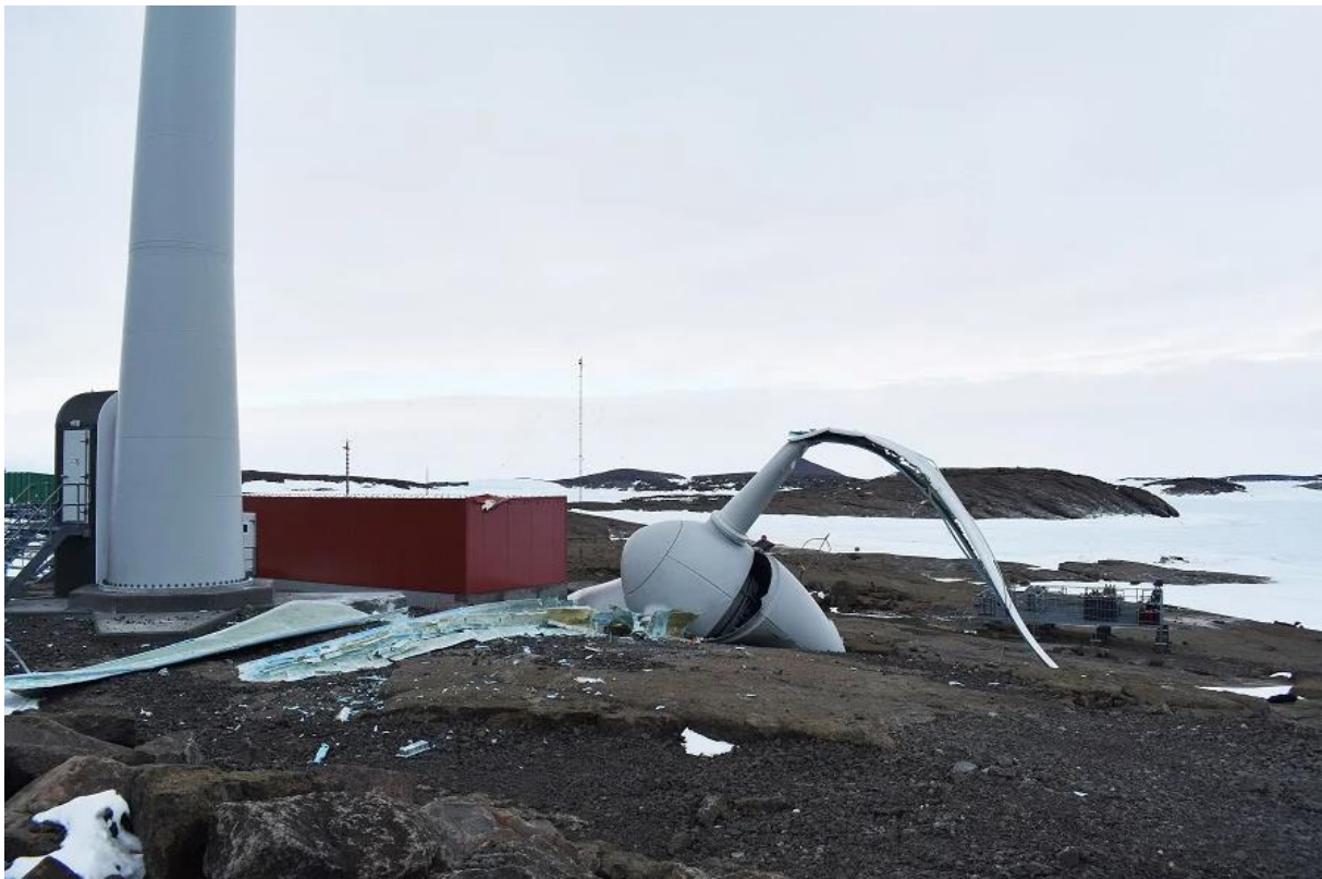
Figure 4-5. Rotor has fallen off a wind turbine in Antarctica, source [Pedestriangroup, 2017]
