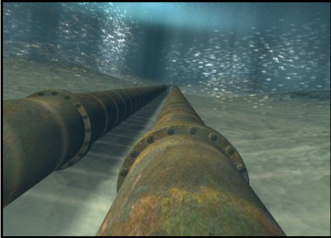
Figure 7 Corrosion of iron [13]
