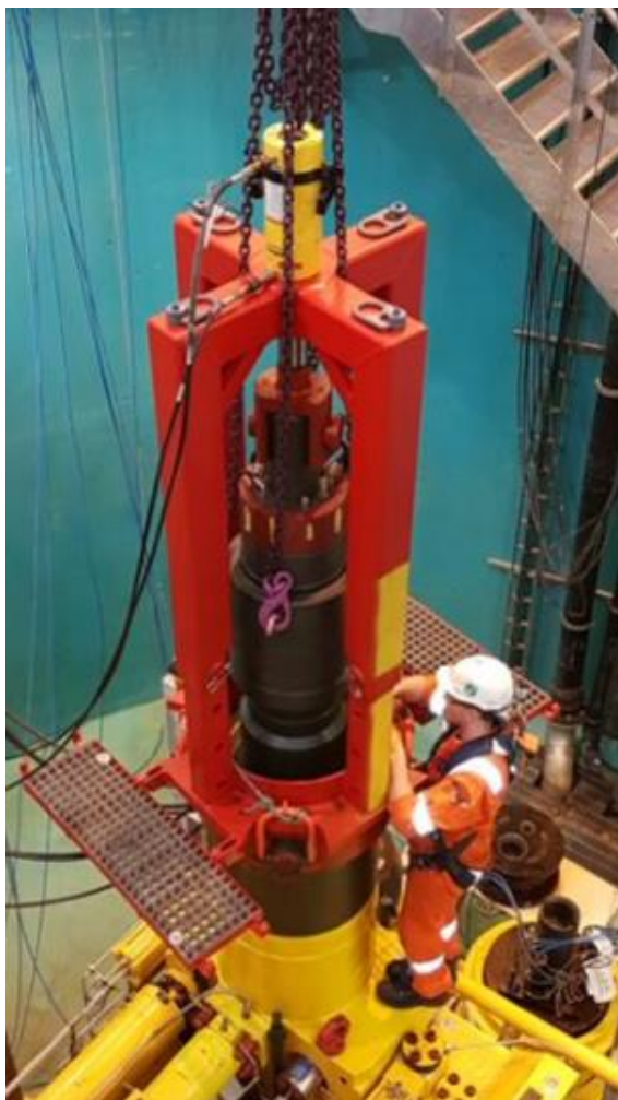
Figure 9 & 10: Rioperk installing TH on top of XT & drawing of installation process [25].
