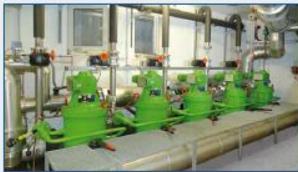
Fig. 3 river water filtration for cooling plant
