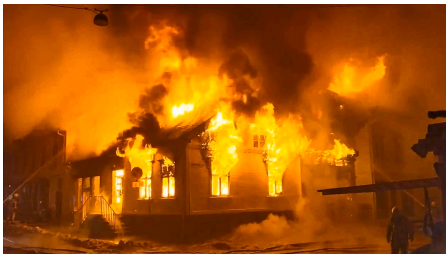
Fig. 10. Fully developed (post flashover) fire in the first building involved 24 February 2014, Risør historical village, Norway. (Photo by Hans Petter Bjerva. Reproduced with permission).
