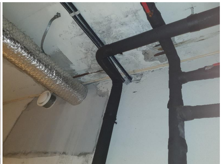
Figur 406, Synleg armering i bassengkjellar, plan 0
