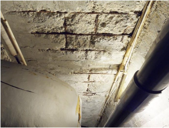
Figur 407 Synleg armering i dekke under basseng, plan 0
