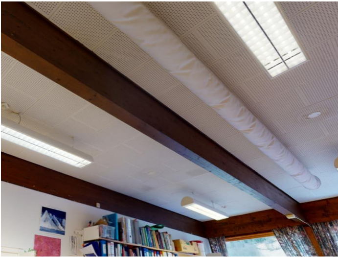
Figur 139 Synlege limtrebjelkar i plan 1
