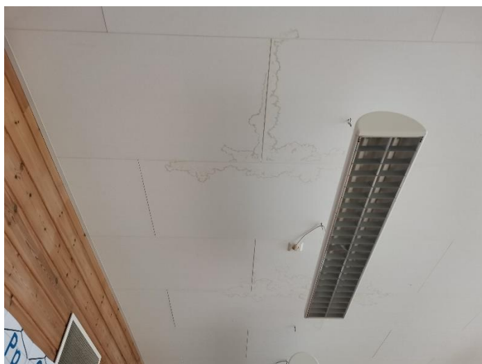
Figur 230 Himling fuktskade
