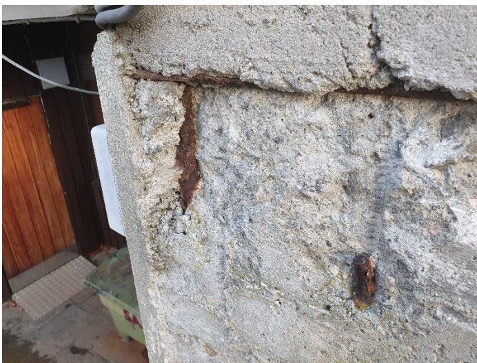
Figur 105 Betongvegg synleg armering, plan 0
