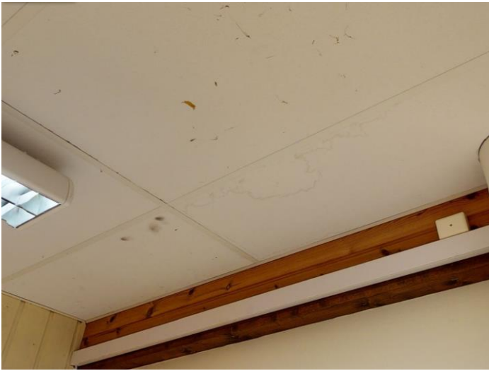
Figur 309 Himling fuktskade
