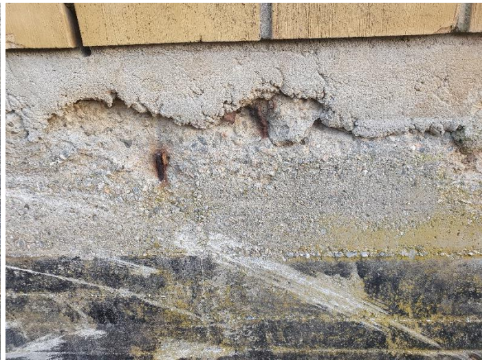
Figur 104 Betongvegg synleg armering, plan 0
