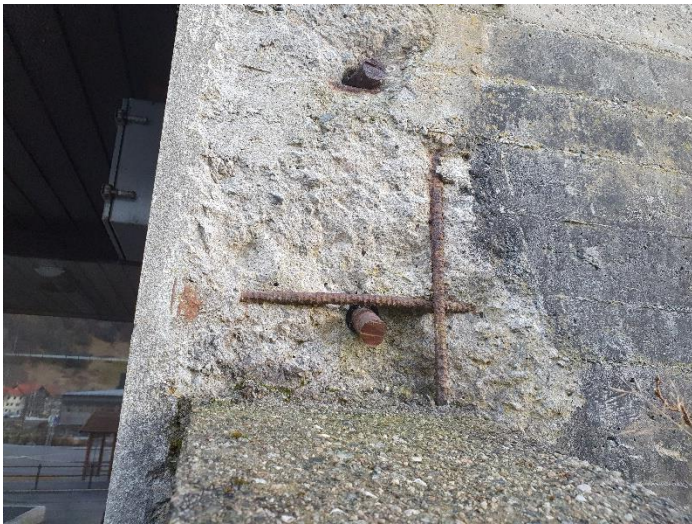
Figur 103 Betongvegg synleg armering, plan 0
