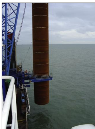
Figure 3: Monopile stabbing [19]
