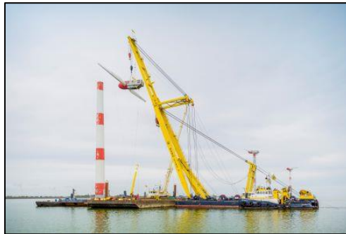
Figure 20: Rotor lift Lely [51]
