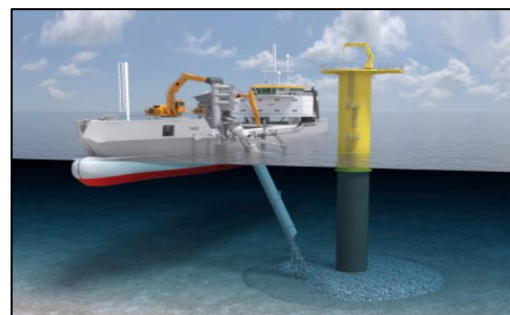
Figure 5: Rock dumping [22]
