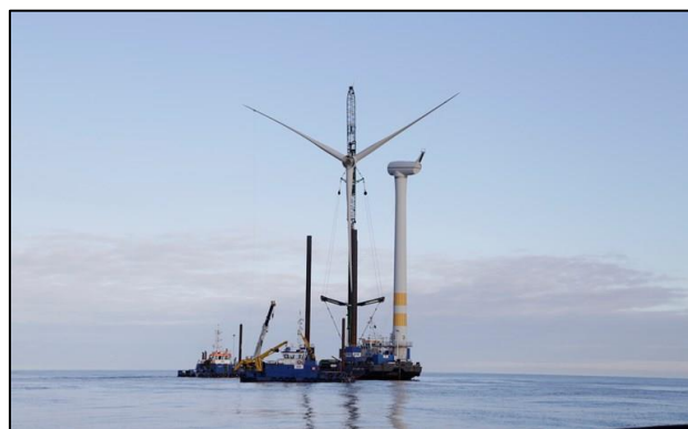
Figure 19: Rotor lift Stengrund [50]
