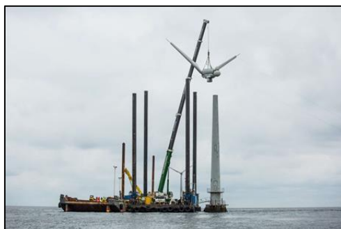
Figure 21: Rotor lift Vindeby [52]
