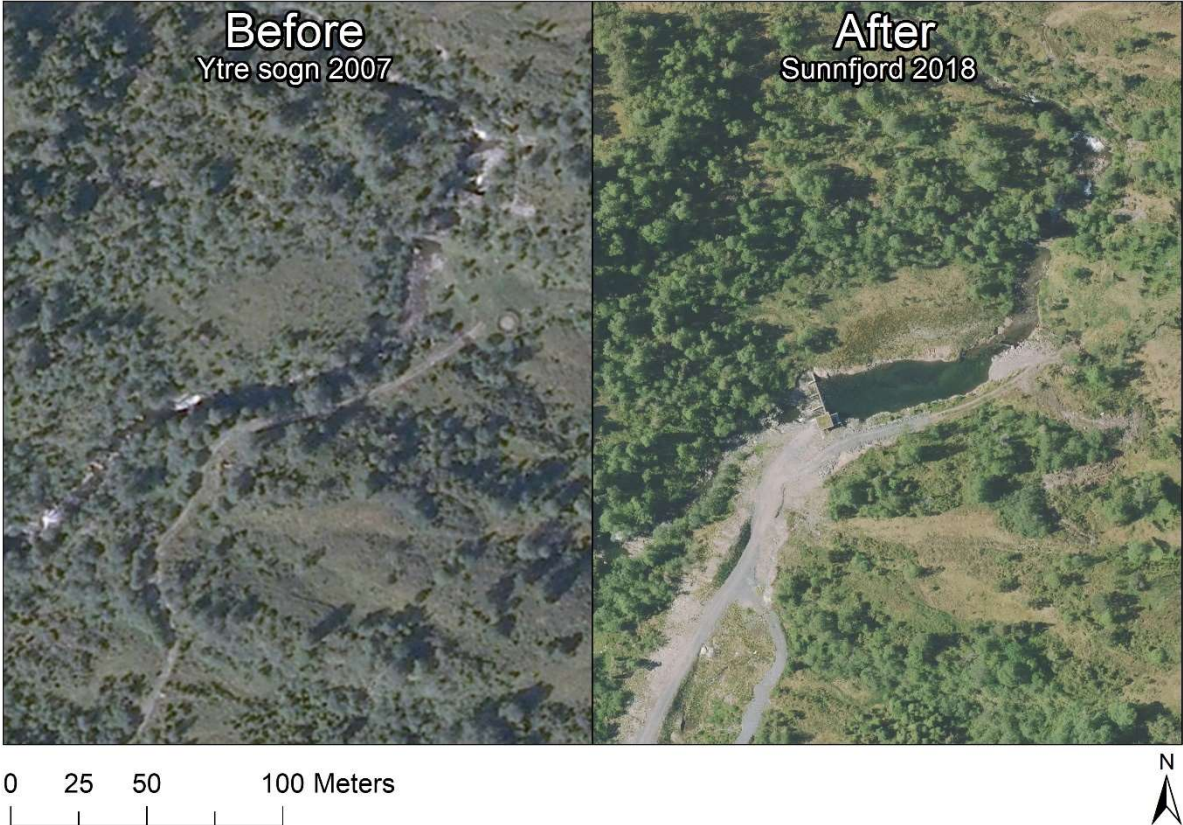
Figure 9: The intake at Kvamselva power plant uses 2 daa temporary area and 1 daa permanent area according to the concession application. The dam has noticeable effect on the amount of water downstream. Images collected from norgeibilder.no. The caption on the figure refer to the layers used from norgeibilder.no, Ytre Sogn 2007 and Sunnfjord 2018. Ytre Sogn and Sunnfjord refers to the area covered of the layer and 2007 and 2018 refers to the year the aerial photographs were collected.
