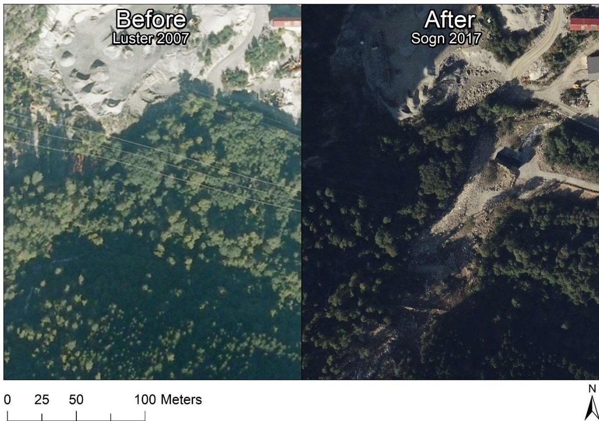
Figure 19: The powerhouse at Røneid power plant is situated in the near proximity of a quarry. The effect of this is that the powerhouse itself doesn't add much to the negative impact of the area. The application estimates that the powerhouse will use 0,2 daa. Images collected from norgebilder.no. The caption on the figure refers to the layers from norgebilder.no and is the name of the layers containing the aerial photos. The first part of the caption refers to the area contained in the layer and the last part refers to the year the aerial photos was created i.e. Sogn 2018 contains aerial photos from the area of Sogn from 2018.
