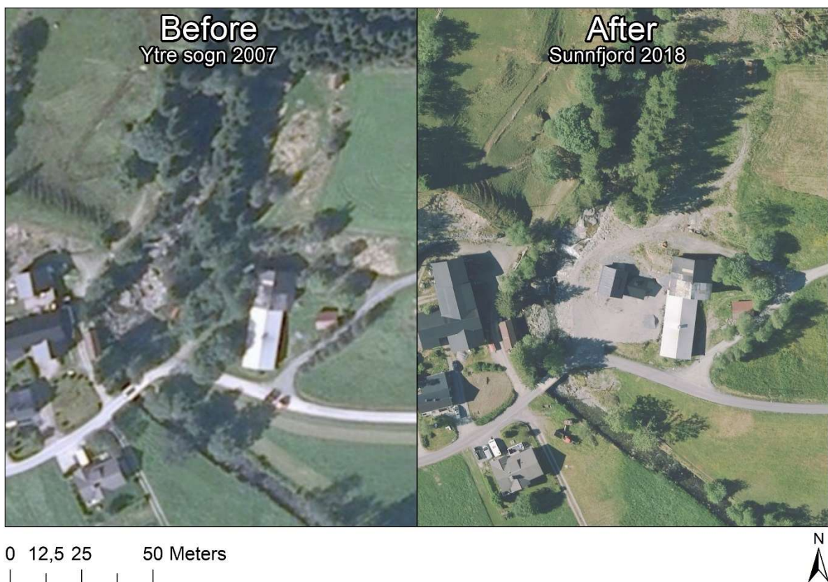
Figure 10: At Kvamselva power plant the powerhouse uses 1 daa in temporary area while 0,5 daa in permanent area according to the application. The powerhouse contains a 2,67MW pelton turbine. Images collected from norgeibilder.no. The caption on the figure refer to the layers used from norgeibilder.no, Ytre Sogn 2007 and Sunnfjord 2018. Ytre Sogn and Sunnfjord refers to the area covered of the layer and 2007 and 2018 refers to the year the aerial photographs were collected.
