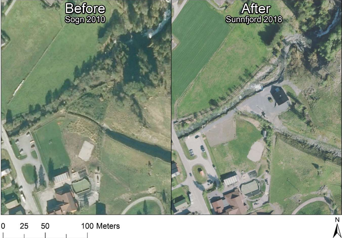
Figure 7: The powerhouse for Holsen power plant is located 451 meters below the intake. The powerhouse contains one 8,6 Pelton turbine. The application estimates that the powerhouse uses 1,2 daa in permanent area and 2 daa in temporary area. Images collected from norgeibilder.no. The caption in the image Sogn 2010 and Sunnfjord 2018 refers to the layers from norgeibilder.no used in the relevant image. Sogn and Sunnfjord refers to the area which is available in the relevant layer while 2010 and 2018 refers to the year the aerial images were taken.
