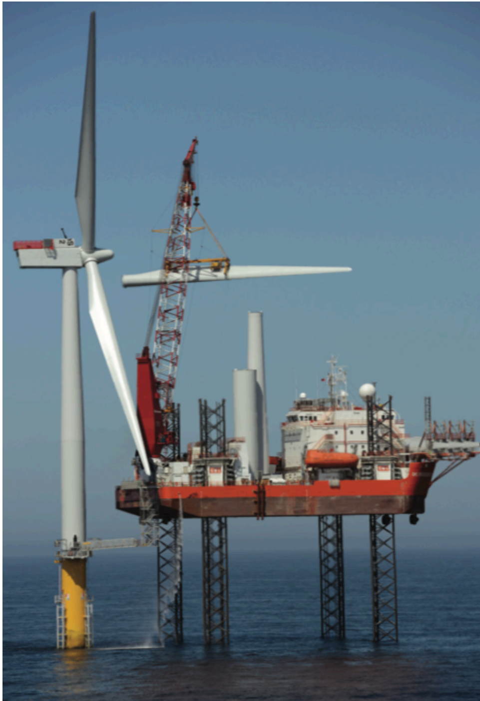
Figure 7 Mounting of blades at Sheringham Shoal using jack up vessel. [6]
