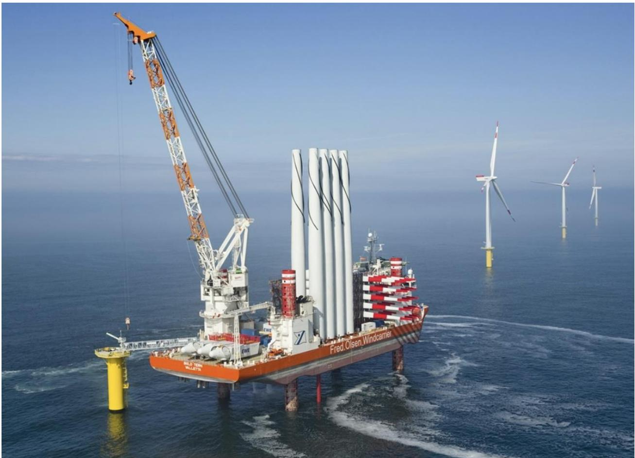
*Figure 8: Fred. Olsen Windcarrier installing monopile, fixed-bottom OWT [13].*
