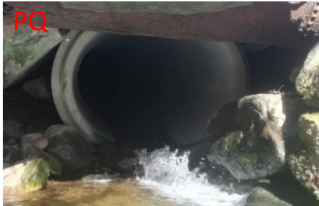
Figure 17: Pictures of PQ2, PQ5 and PQ6 show the three pipe outlets of the municipality stormwater management system. Photos taken by Tewelde Mebrahtu Tesfay.
