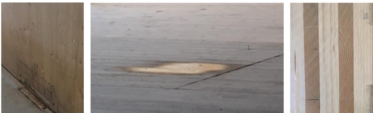
Figure 44 Observed high-risk locations in the Skipet project; CLT-Concrete connections, covered stains and gaps. No significant damage is found [by author]
