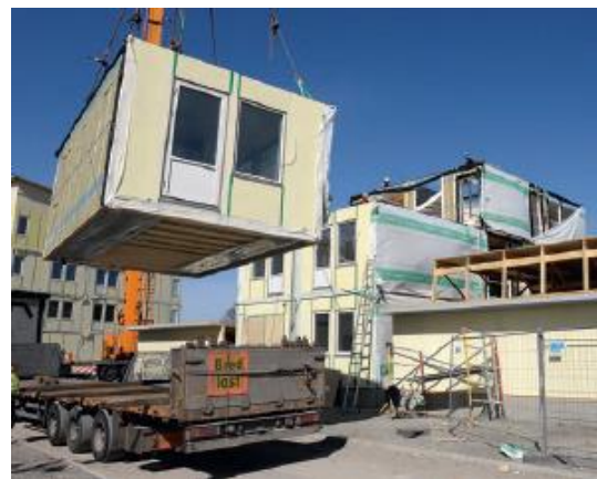
Figure 11 CLT modular system [11]
