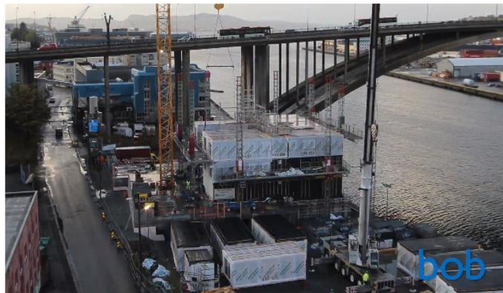
Figure 50 Construction site of the Treet project. Installation of the prefabricated modules [62]
