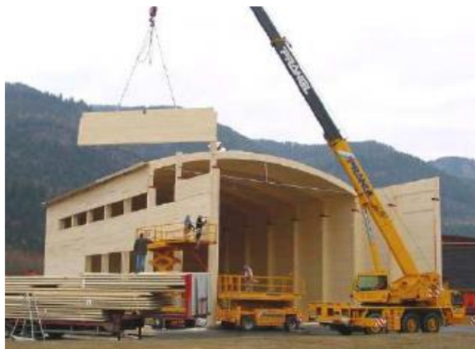
Figure 22 CLT prefabrication and on-site assembly [26]
