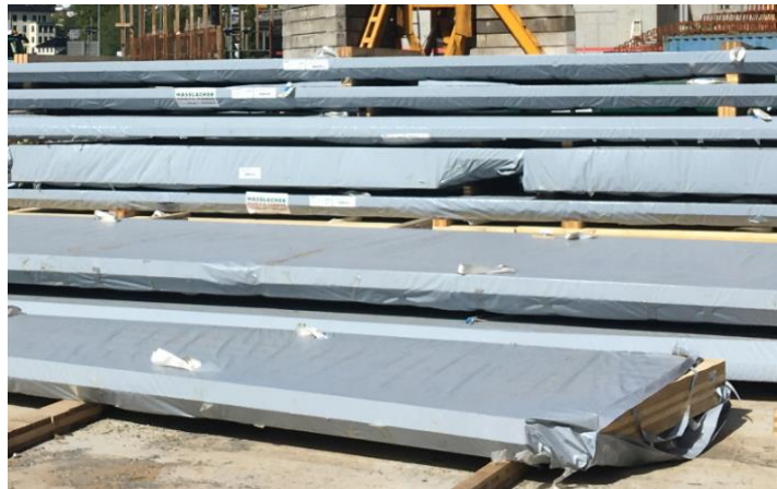
Figure 37 On-site storage of manufacturers' sealed CLT elements – Project: Skipet [by author]
