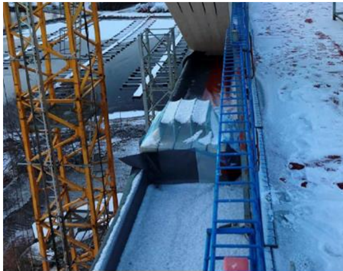
Figure 48 Plastic covers as end-grains protection [30]
